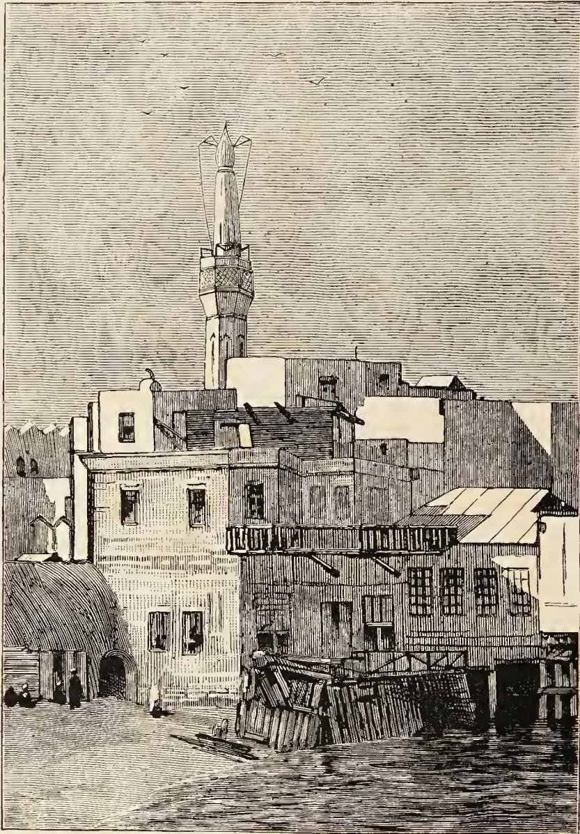
HOUSES AT THE OLD PORT, ALEXANDRIA.
